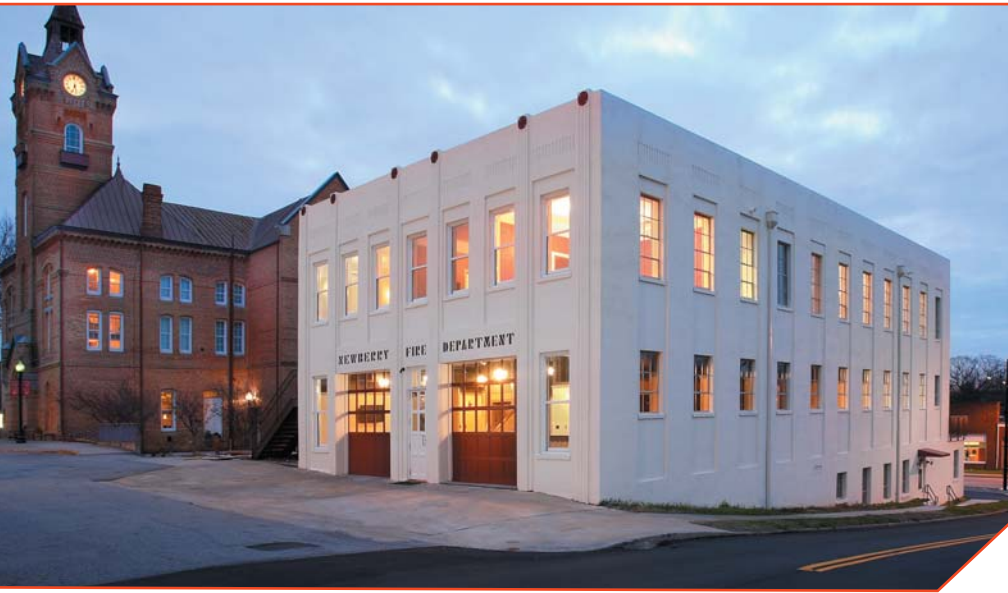
The Newberry Fire House Conference Center draws residents and visitors downtown for meetings, training, weddings and other social events. (Photo/city of Newberry)
