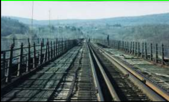
Poughkeepsie High Bridge - Before
