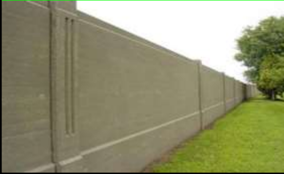
Paducah Flood Wall – Before
