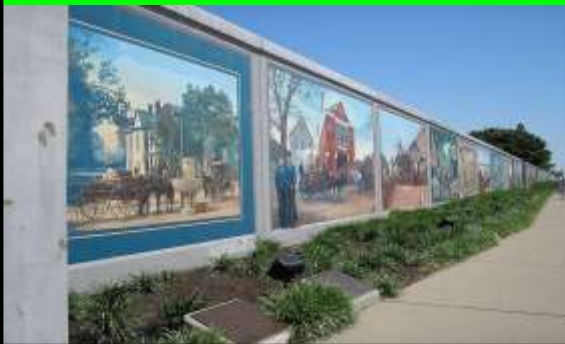
Paducah Flood Wall - After
