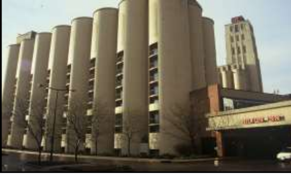
Akron Grain Elevators - After
